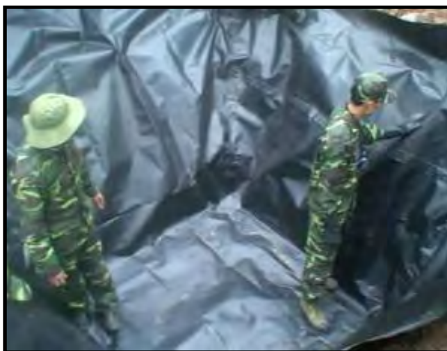
Photo 1: Burial pit lined with impermeable plastic sheet.
