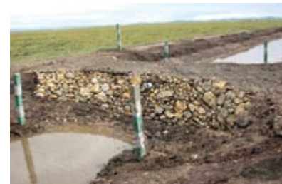
Dams construction for rewetting. Photo: Zhang Xiaohong
