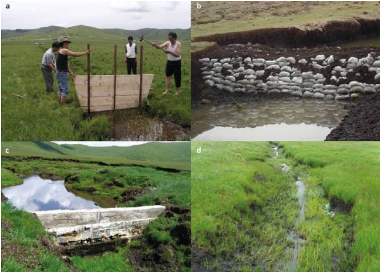
Peatland restoration. Blocking canals by a: wood plank; b: peat; c: concrete damming; and d: revegetation
