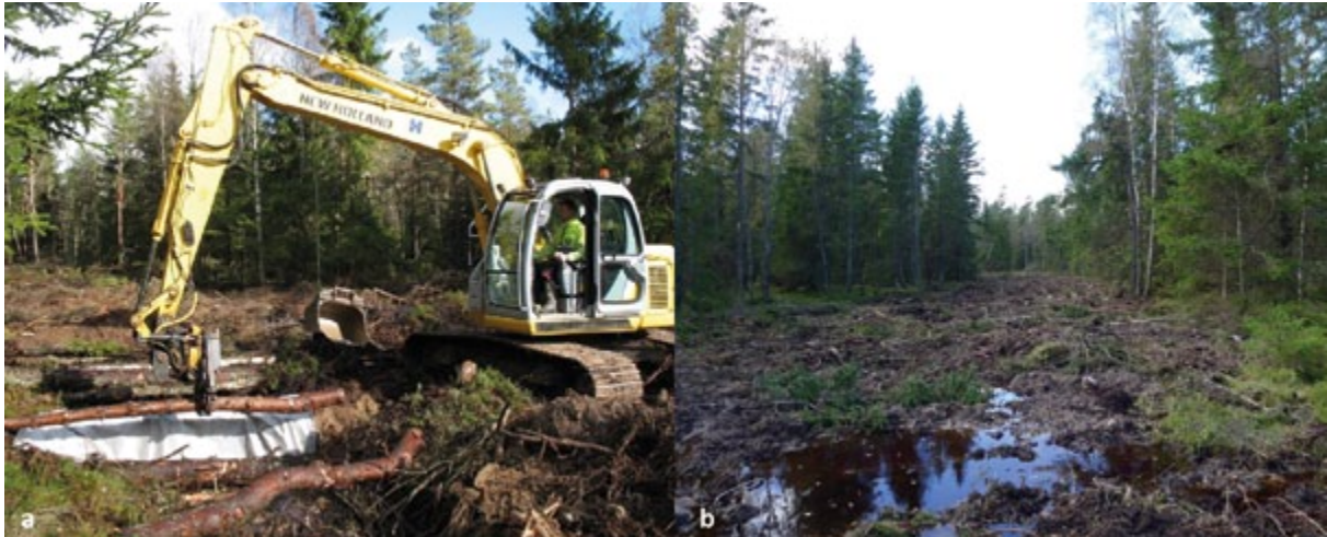
Rewetting the peatland a: Excavator building dams and filling ditches in drained fens and wet forest and b: rewetted site immediately after the completed restoration actions.
