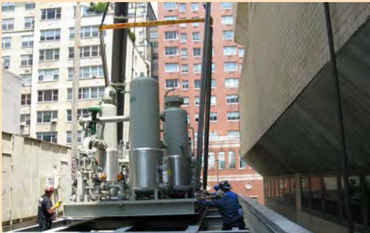
Gas compressor installed as part of New York-Presbyterian Hospital's Combined Heat and Power system. (Credit: New York-Presbyterian Hospital)
