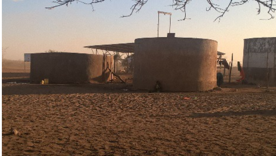
Figure 3: A concrete water tank in Shurr (Source: IUCN 2016)
