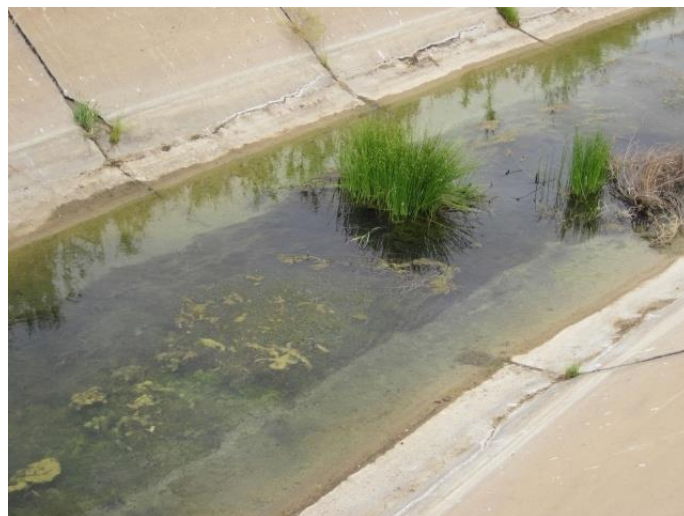
Plate 5 Water conductivity is much higher in agricultural return flow channels than in the main river channel, favouring different blackfly species
