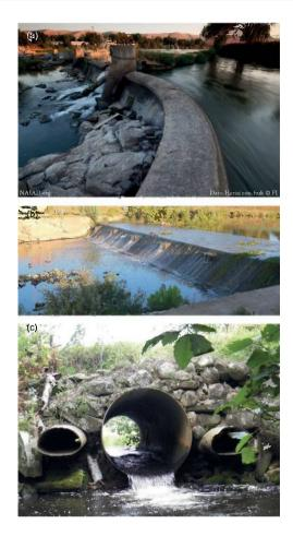
**FIGURE 1** Examples of small instream infrastructure: (a) dam, (b) weir, and (c) culvert that were the focus in reviewed studies. Shown are a low head diversion dam on Yakima River, Washington, D.C. (photo by David Herasimtschuk); a weir on Lez River, France (photo by Stephanie Januchowski-Hartley); and a culvert at the intersection of a road and stream in Chequamegon-Nicolet National Forest, USA (photo by Dale Higgins)
