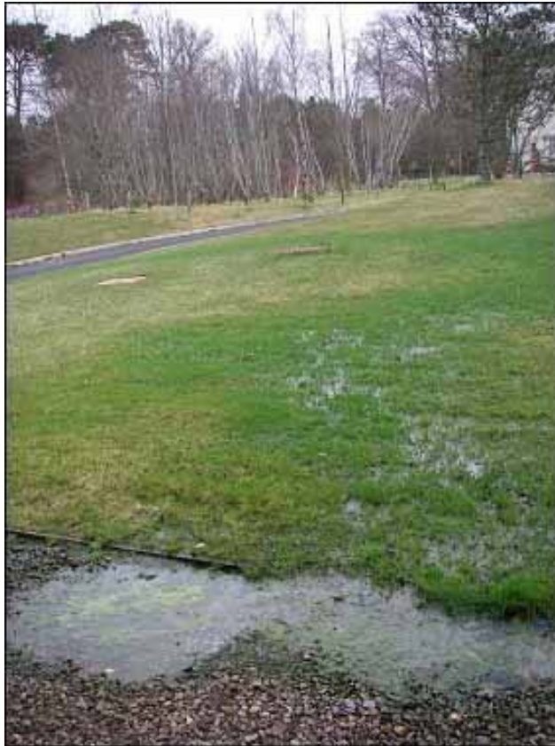
Figure 2.4 Effluent discharging onto the soil surface as a result of hydraulic failure in a septic tank system; note the algal bloom that is developing on the nutrient rich puddle that is forming at the base of the slope.
