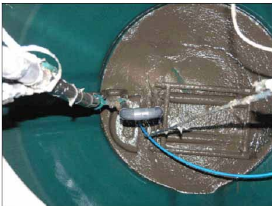
Figure 2.2 Floating scum layer inside the reactor vessel of a 'Balmoral' septic tank as viewed from above. The tubing forms part of the "air lift" pump system that transfers effluent between the chambers and pumps clarified effluent out of the system (Image courtesy of J Malley, National Trust).
