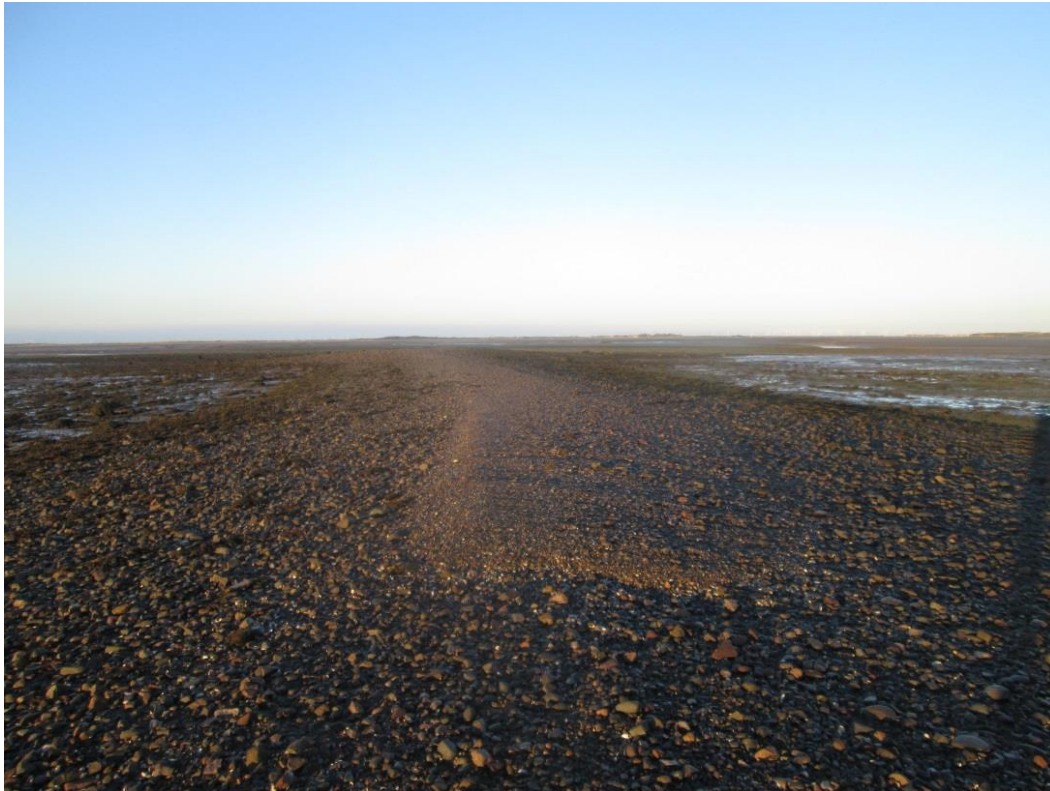
Figure 9 Raised shingle bank which is mainly barren offshore from Roosecote Power Station.
